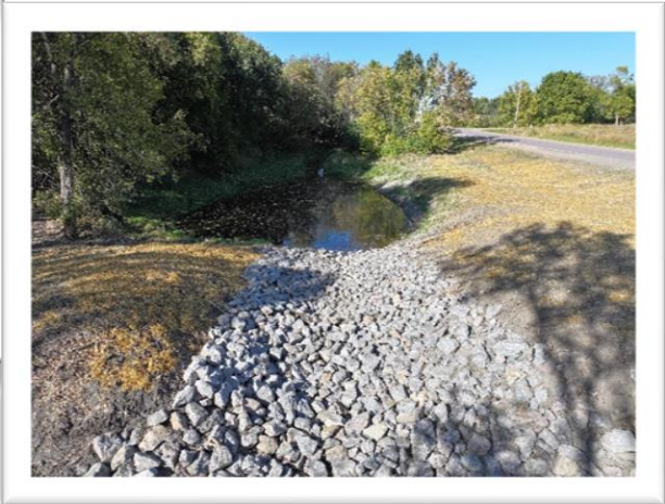
After - Completed Project
