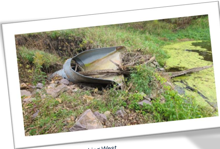
Before - Upstream looking West
